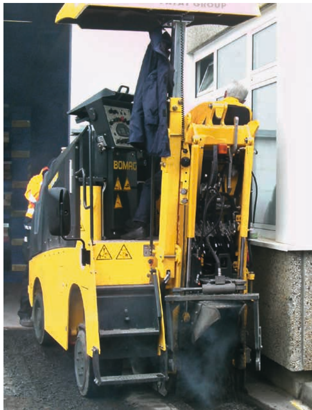
Precise working close up to the house wall? No problem.
